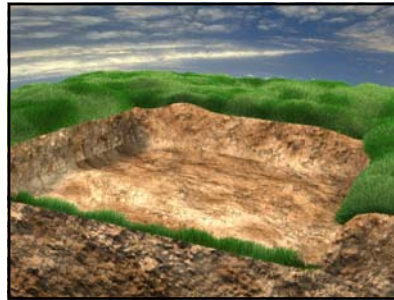
7" to 12" soil excavation depending on application
